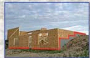
Prevent dust and moisture entry through plate lines.
