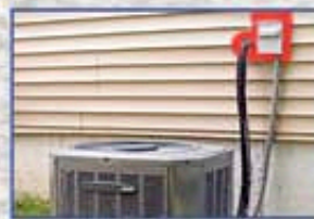
Seal air conditioning penetrations.
