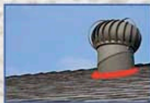
Close leaky gaps in attics and roofs.
