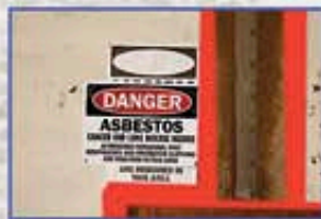
Positive air sealing in asbestos removal areas.
