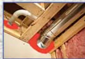
Seal utility penetrations.
