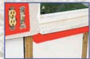
Stop air infiltration through windows, electrical outlets.
